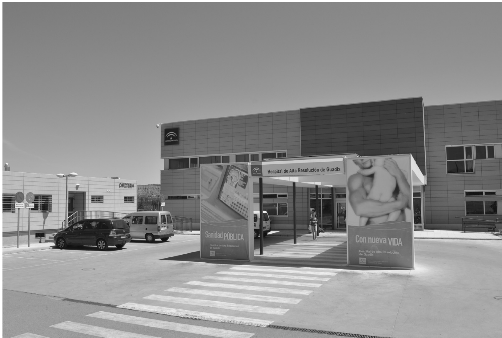
Entrada principal del Hospital de Guadix. RAMÓN UBRIC.
