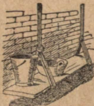
Scaffolding. Scáfolding. Un andamio.
