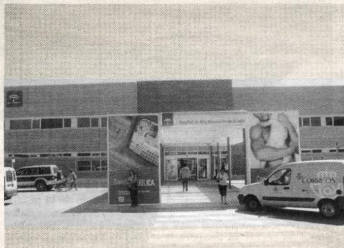
Hospital de Guadix.
