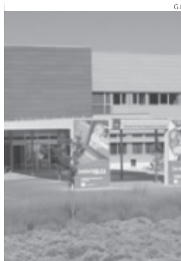
Hospital de Guadix.
