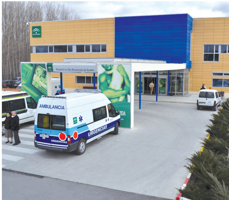
Hospital de Guadix.
